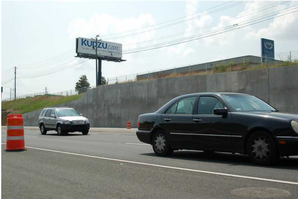
Figure 2 After view of Mercedes dealership from road showing 30 foot retaining wall introduced to show change in visibility and access
